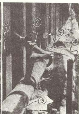
図-4a 名鉄 Well point
