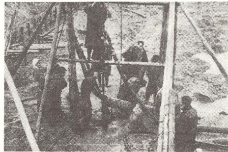
図—16 庭窪 Well point の jetting test
